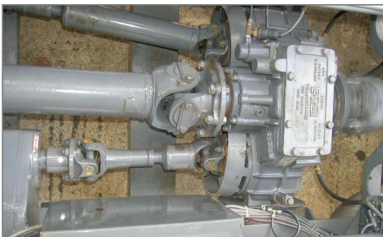
Split-shaft PTO driving of vacuum pump and Hi-pressure water pump.
