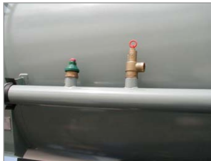
Vacuum and pressure relief valves protect the systems
