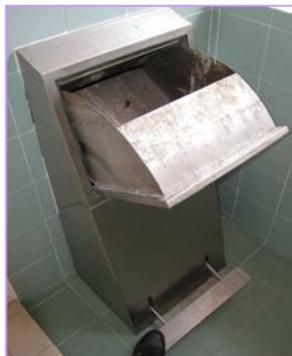
Residents throw their refuse into the above "fixed-volume" foot-operated stainless steel hopper. The hopper is designed such that no bulky refuse is thrown into the chute (probably only 3 or 4 average-sized telephone directories can fit into the hopper).
